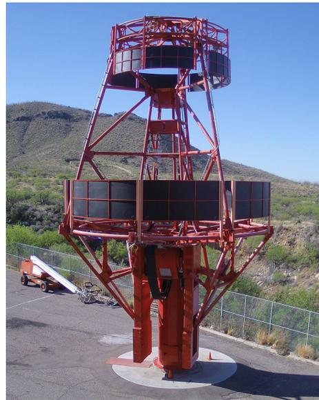
*The construction of the mechanical system of the Schwarzschild-Couder Telescope prototype at the Fred Lawrence Whipple Observatory in Arizona. Credit: CTA*
